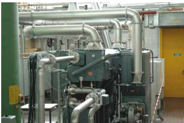
Trigeneration: an absorption chilling system charged with hot exhaust gases from micro turbines for a distributed and environment-friendly energy supply for an island in the Caribbean. Institute of Thermal Turbomachinery in cooperation with the European Institute for Energy Research (EIER)
